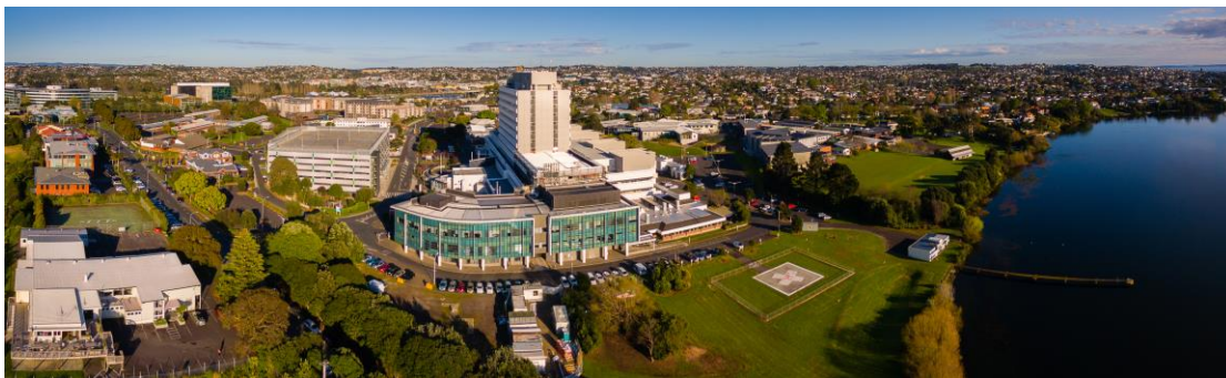
North Shore Hospital
