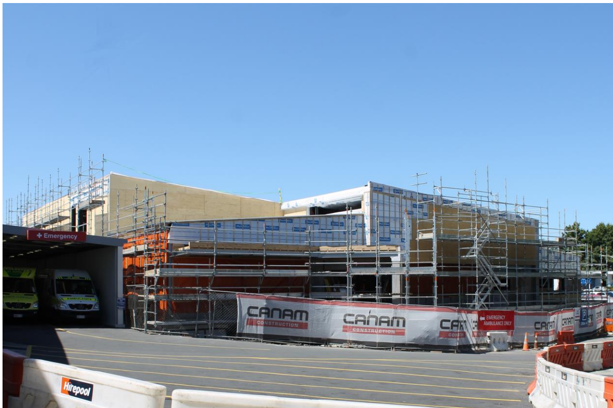
Waitakere Hospital's new emergency department under construction.
