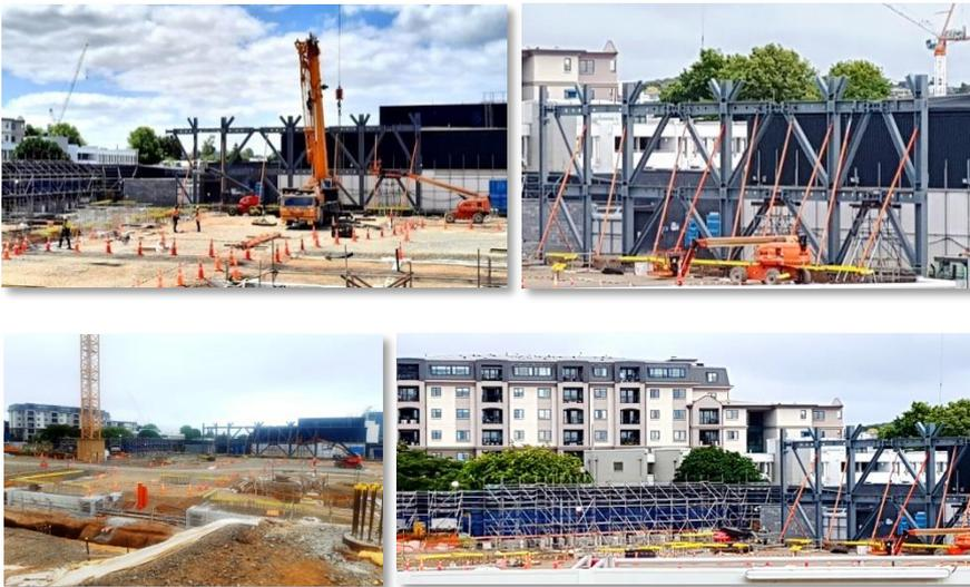
*Seismic k-bracing structural steel being installed on-site*
