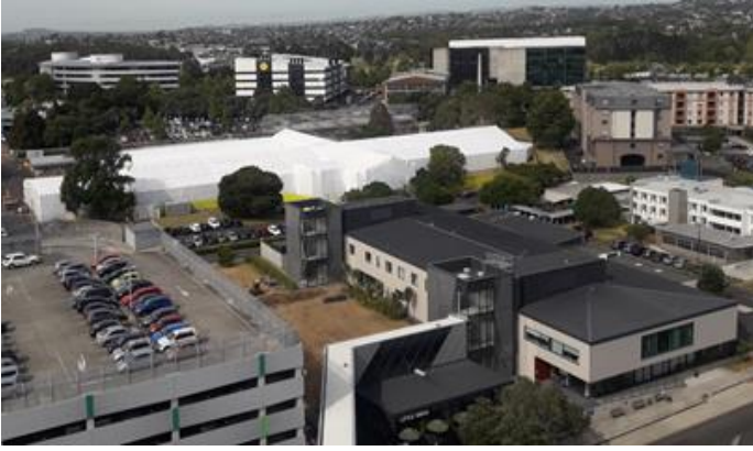
Image of the 'shrink-wrapped' Pupuke & Taharoto Buildings taken from the North Shore Hospital Tower.
