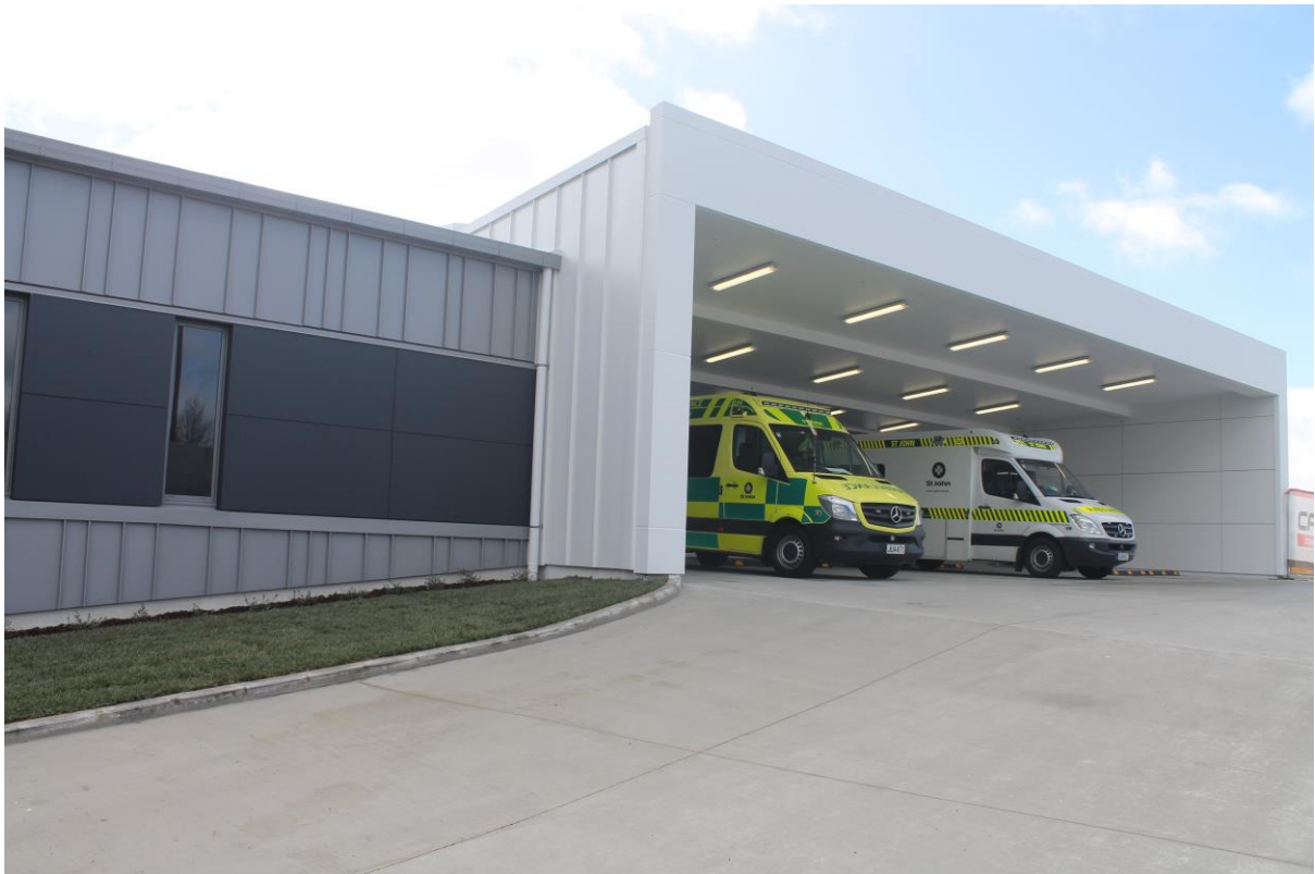
Waitakere Hospital Emergency Department Ambulance Bay
